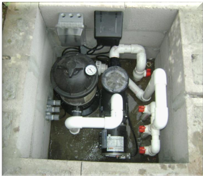
New Equipment Installation In Ground Vault
